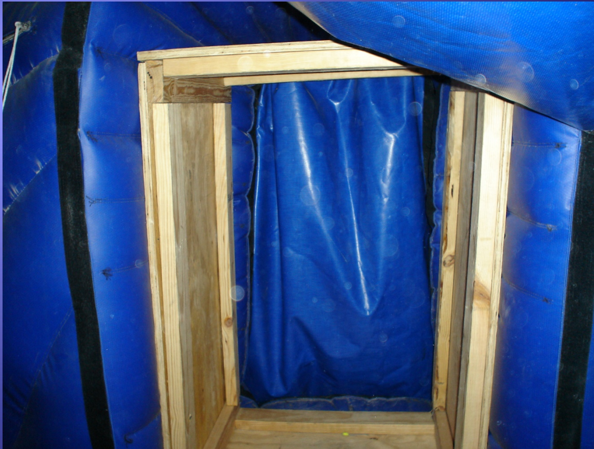
Wooden liner for 6 x 3' access door
